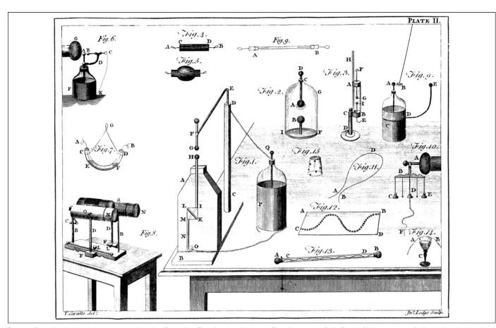
Figure 1. Portable electrical instruments used in scientific soirées. Fig. 1 is a thunder-house, Fig. 2 is an aurora flask, Fig. 8 a friction generator (cylinder electrical machine), Fig. 10 electric bells, Fig. 12 a magic board, Fig. 13 a luminous tube. From Tiberius Cavallo (1795) A treatise on electricity, London. Courtesy of the Bakken Library and Museum for Electricity in Life.
