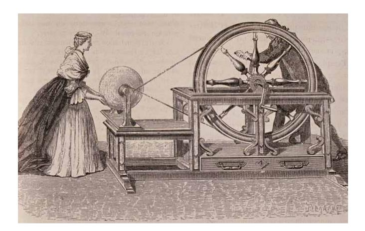
Fig. 6. Electrical machine (Nollet 1746).
